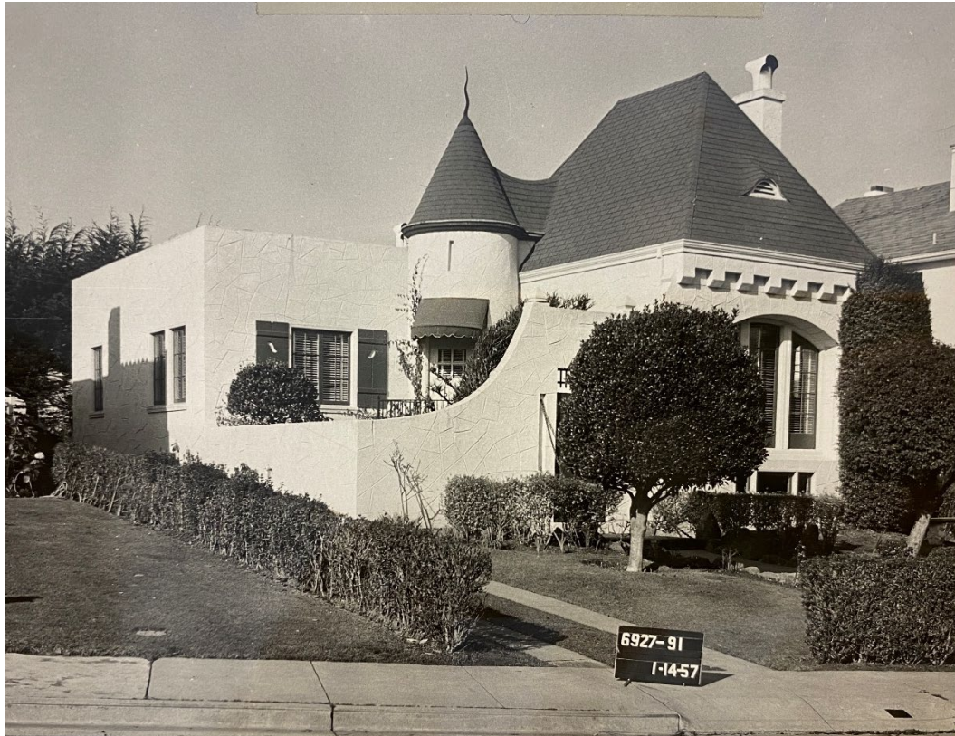
Figure 13 91 Borica Street (Resource #64, built 1923), shown in 1957. Source: San Francisco Assessor-Recorder Collection, San Francisco Public Library.
