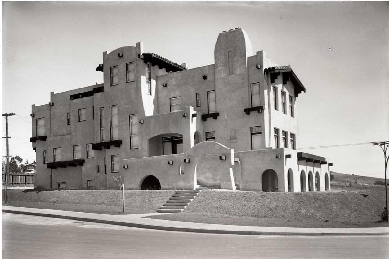
Figure 8 145 Paloma Avenue (Resource #596, built 1913), circa 1915. Source: San Francisco History Center, San Francisco Public Library, SFP22-0130.
